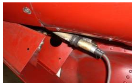
Pump return line installed in the blow-by port (in a Mooney 231).
