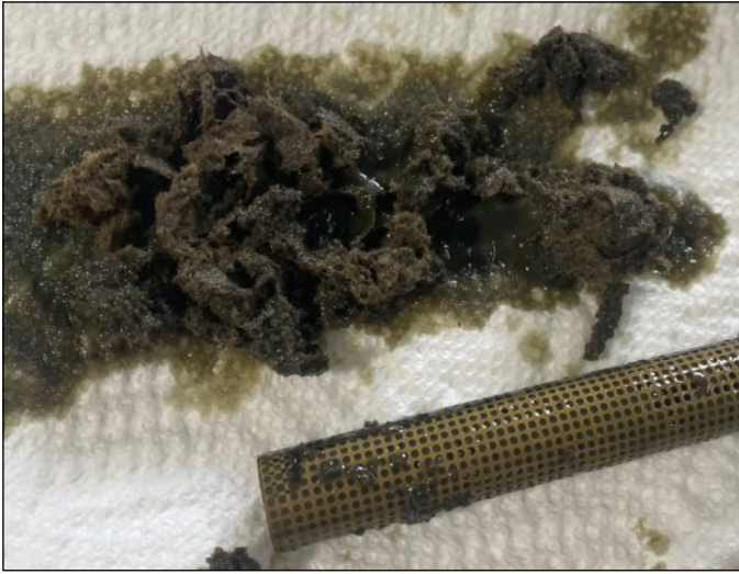
Fig. 5: After we pried the debris out
